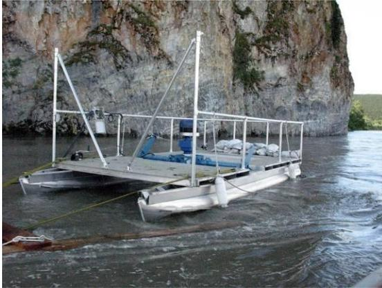
The installation of the pontoon boat was carried out by first installing the boom deflector. Then the pontoon boat was moved into position by tying it off to a second boat which then maneuvered it to a position downstream of the boom deflector. Once in position downstream, it was motored into position directly behind the boom deflector and attached to the buoy
